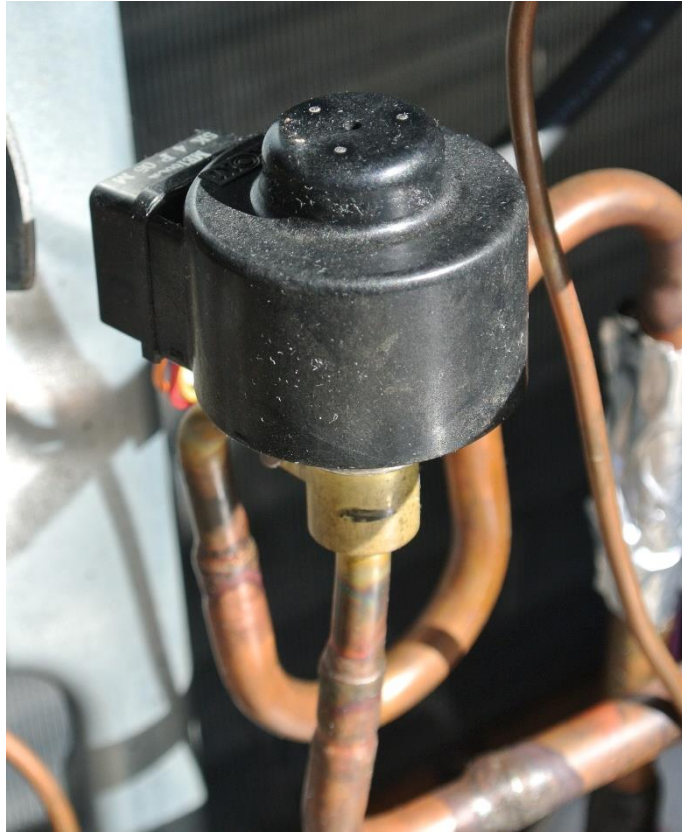
Figure 2.4 Picture of expansion valve
