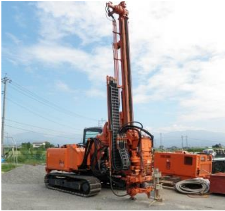
Figure 2.13 Picture of sonic drill
