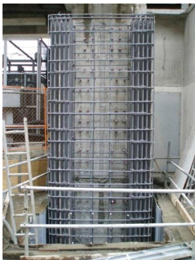
図-6.25 鉄筋組立て
