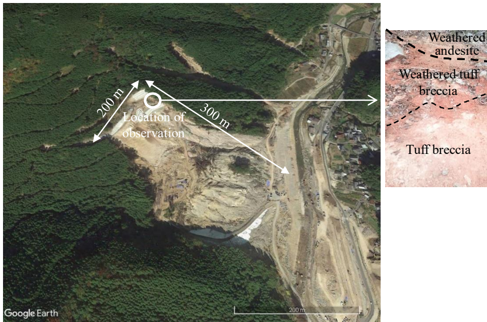
Photo 4.8 Ono landslide and soil materials in the landslide (Taken on July 2017) in length and 200 m in width, furthermore, two collapses occurred in the Ono landslide; andesite was exposed in the lower collapse and weathered tuff breccia was exposed in the upper collapse (Photo 4.8). Similar to the Ohtsuru landslide, Ono landslide was divided into 3 sub-layers; consists of weathered andesite, weathered tuff breccia, and tuff breccia. Unfortunately, because of the condition of the field which difficult to exposed the soil layers, the depth of the soil layers in the Ono landslide could not be identified.
