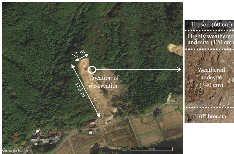
Photo 4.7 Ohtsuru landslide and soil materials in the landslide (Taken on July 2017)
